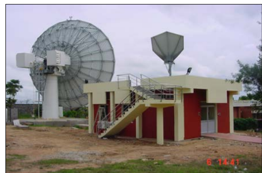
Plate 11. The 13.2m Ka Band antenna at MCF Master Control Facility (MCF), Hassan, Karnataka
