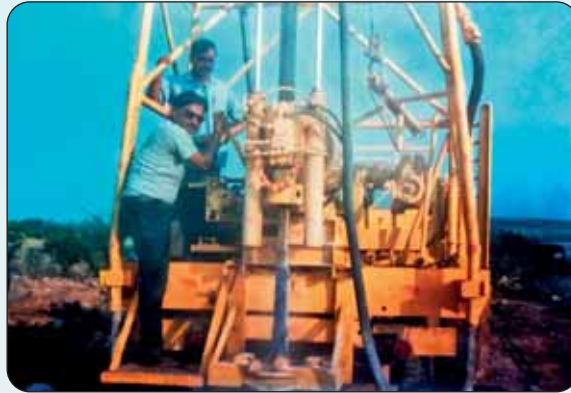
Arjun Prasad operating DL-500 truck-mounted rig
